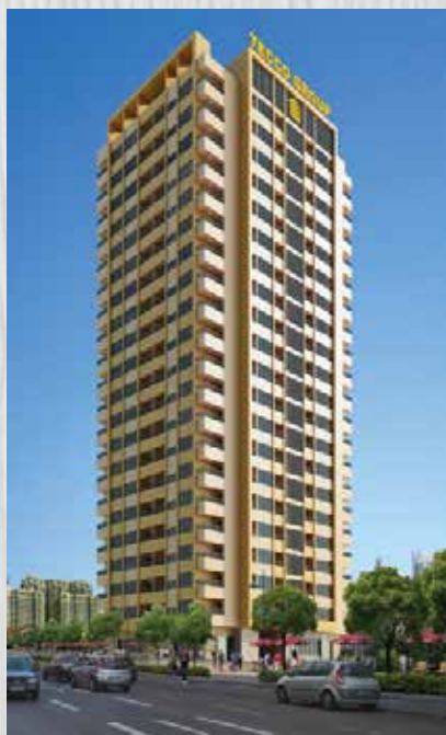
Tecco Binh Duong Project
