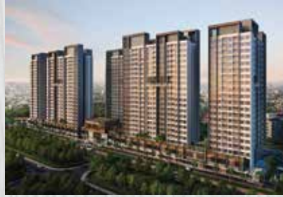
Celesta Project- Phu Loc House
